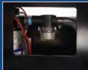
Water System Pump and Filter
