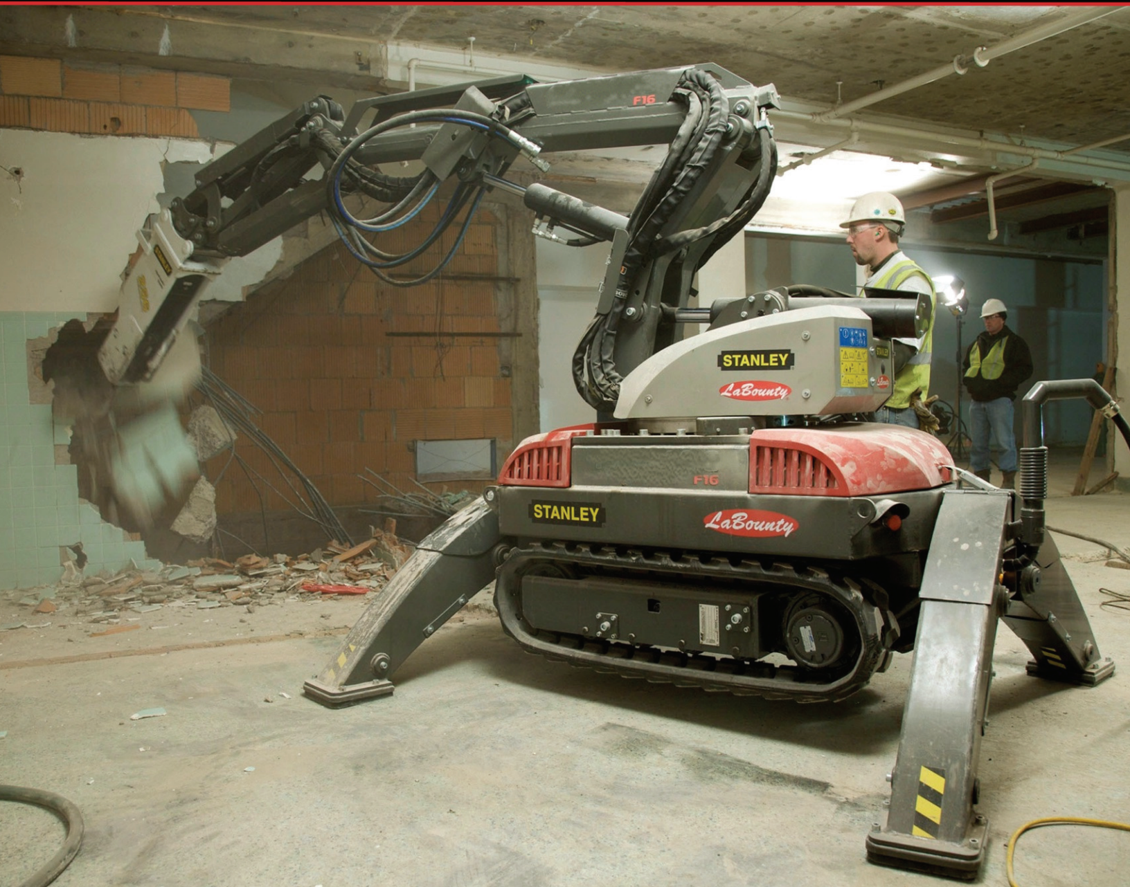
F16 Remote Controlled Demolition Robot
