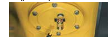
Fuel tank drain valve.
