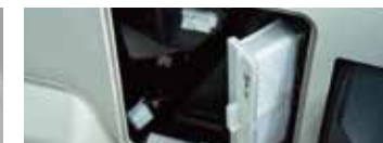
Air Conditioner Filter
